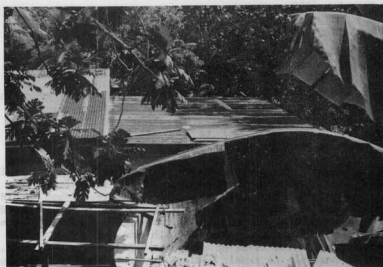
Figure 1. Solar modules mounted on roof of residence in Kuchua Village.
