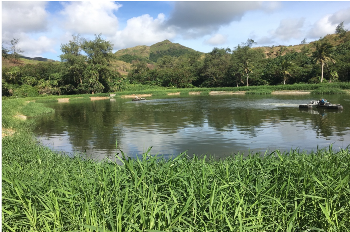
Figure 5. Ponding for cultivating nitrifying bacteria in Umatac-Merizo sewage treatment plant.
