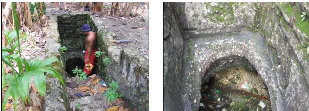
Figure 5. Reef Flat Plate on Mogmog Island, Ulithi Atoll. The residents must punch through the plate to reach the fresh groundwater.
